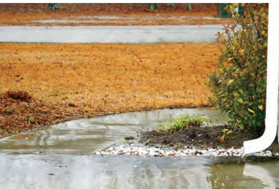
Typical placement of a downspout
